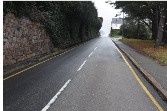
Top of Westmount Road
